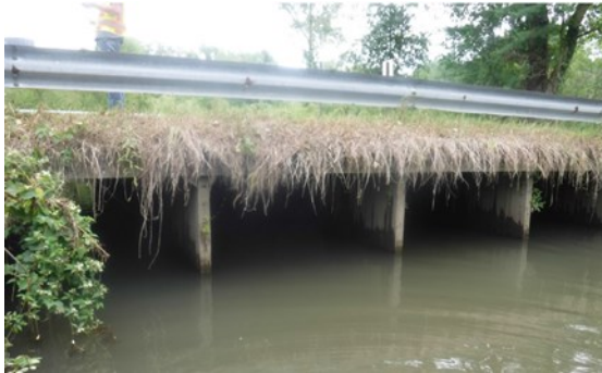
Figure 1: Hill Road over Mill Creek timber culvert
