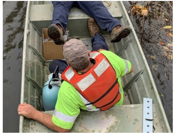
Figure 5: Kurt (BCRD) prior to installing steel plates
