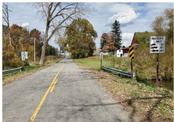
Figure 7: Updated bridge weight limits following repairs
