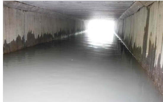
Figure 2: View from inside the Mill Creek timber culvert
