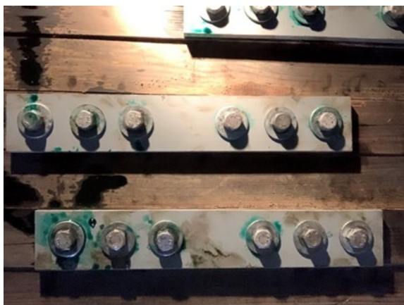
Figure 6: Steel plates installed to timber culvert
