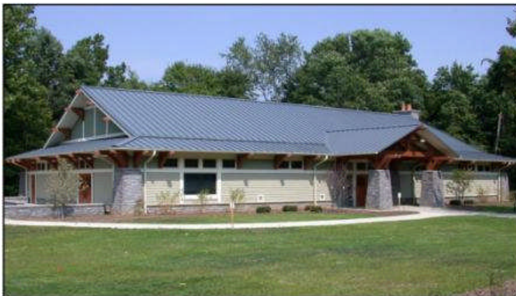
The nature center features program and display areas, as well as observation windows overlooking the Love Creek ravine.
